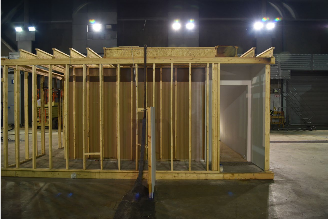
Figure 2. Exterior view of structure (337704_1190276.jpg)
