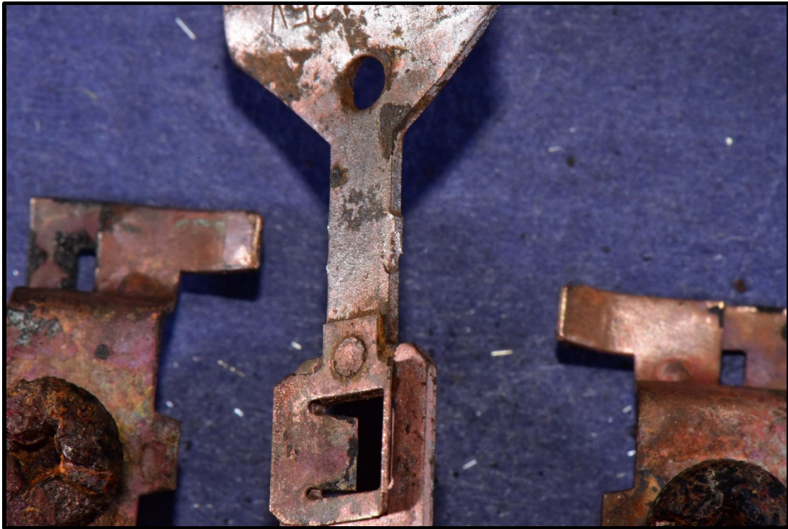
Figure 91. Power rails and ground yoke from Receptacle 11-B
