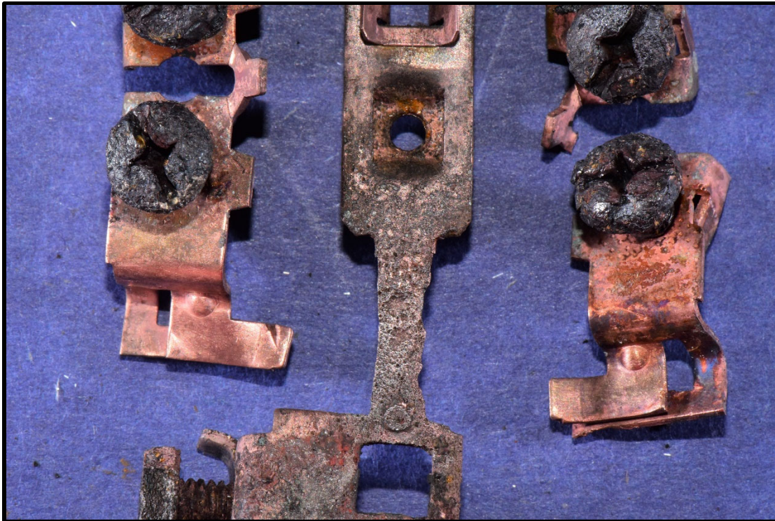
Figure 30. Power rails and ground yoke of Receptacle 11-R
