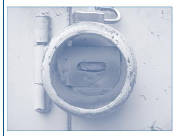
Shallow depth pipes do not prevent prying or lever action on locks.
