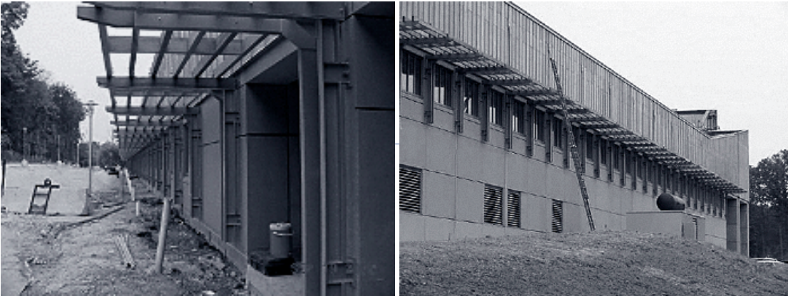
West and east sides of new National Laboratory Center
