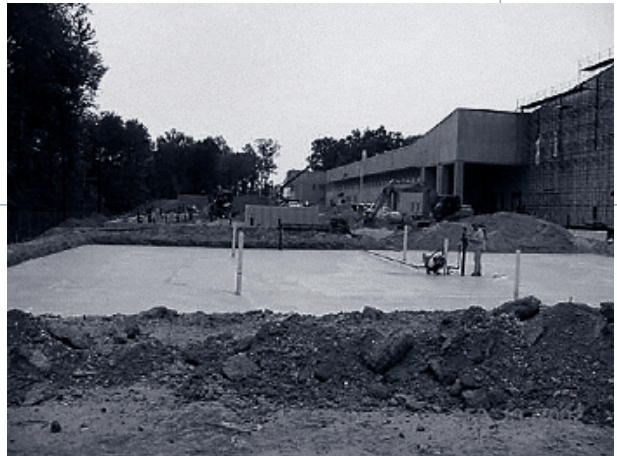
Foundation for the air and water pollution abatement area
