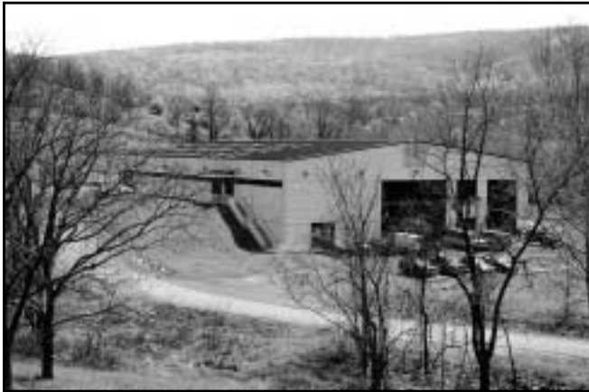
Canine Training Facility in Front Royal, VA.
