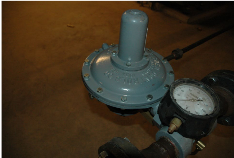
Figure 3 – Type 99 Pressure Reducing Regulator
